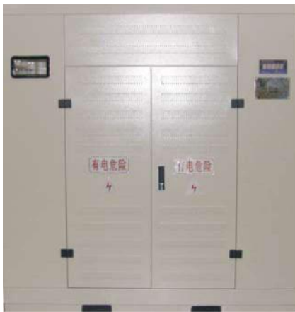
Enclosure of steel plate
